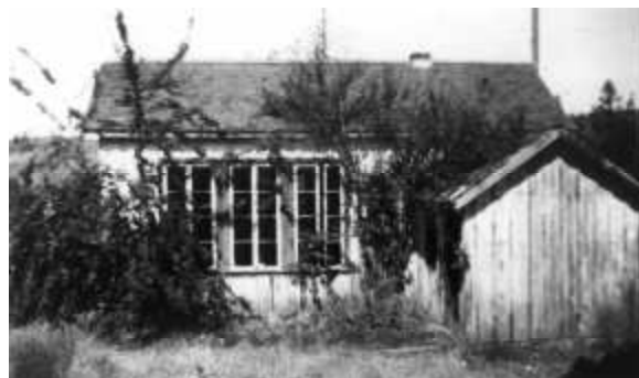
Isabella Point School, 1905–1951, demolished soon after closing
