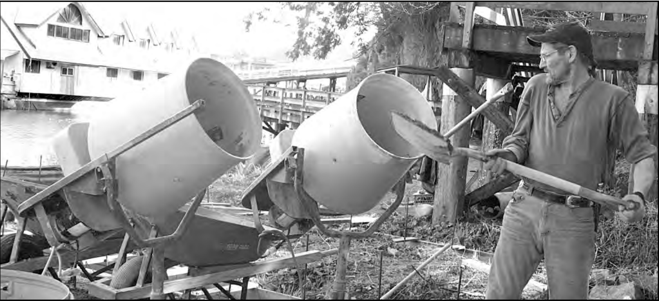
POURING AWAY: The Capital Regional District (CRD) is looking to obtain a court injunction to stop construction of two buildings along Ganges Harbour. Photo by Sean McIntyre
