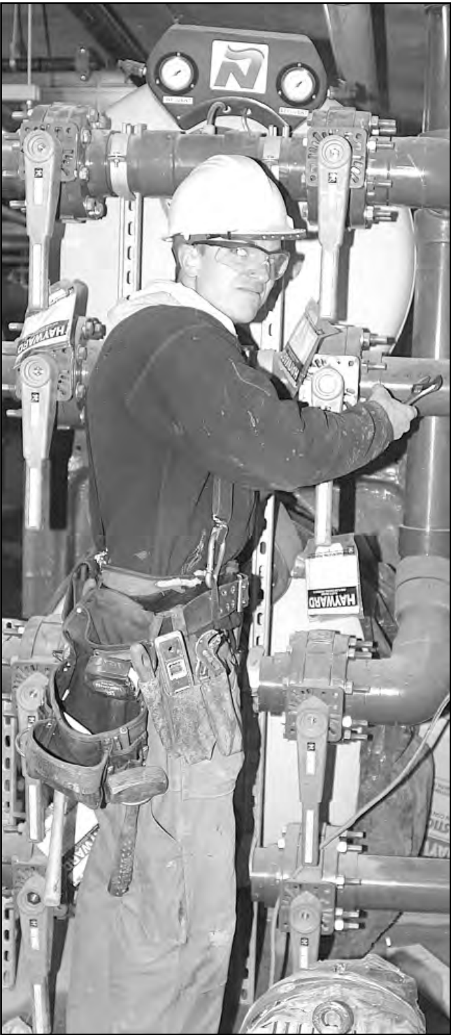
POOL PIPES: Blair Day of Master Pools is seen with the domestic cold water system underneath the Rainbow Road pool facility currently under construction. Photo by Derrick Lundy
