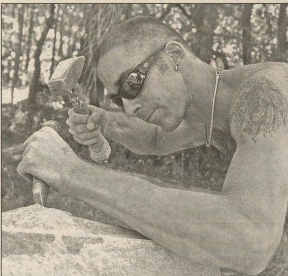
CARVED IN STONE: Stonemason John Heath chisels a stone for a fireplace at a Salt Spring home under construction. Photo by Derrick Lundy
