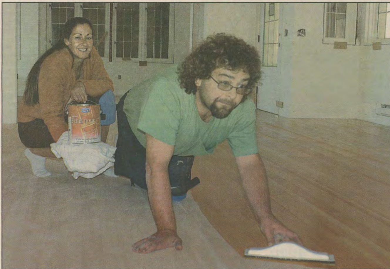
FLOOR SEAL: Johnny Raposo and helper Jill Laird spread a seal coat on a hardwood floor at a Salt Spring home currently under construction. Islanders building or renovating are encouraged to consult first with the island's building inspection office.
