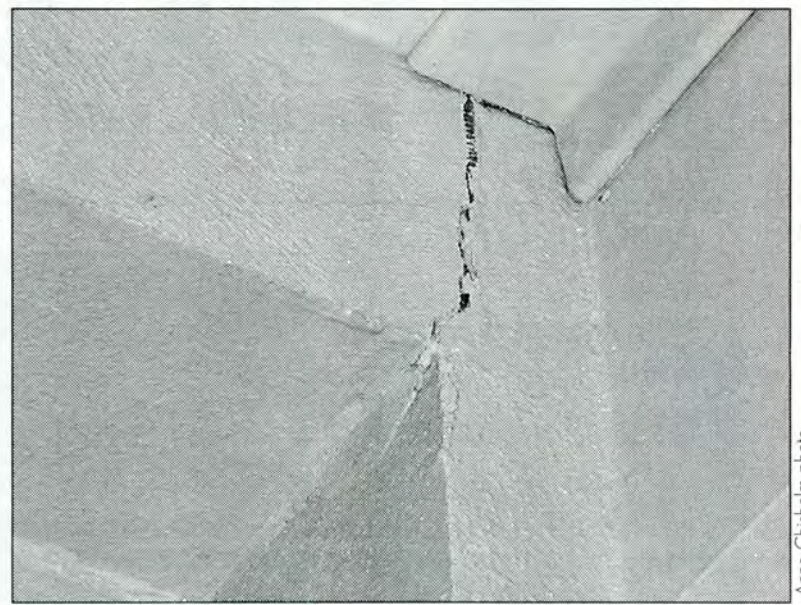
IS IT OR ISN'T IT? —GISS staff were unable to say with any certainty whether or not this crack in a wall in the multi-purpose room appeared or perhaps was increased by last week's earthquake.
